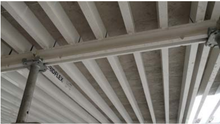
Used instead of the plywood, but 10 times more
