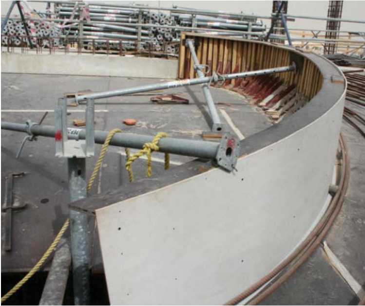
Curved formwork in Shangrilla Hotel construction site - UAE
