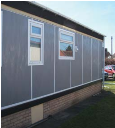
Insulated mobile home, financed by British Gas UK built to illustrate the energy saving potential of Novaplak insulated sandwich panels.
